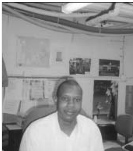
Exposed pipes and electrical wires above union member Albert Robinson’s desk, indicates some problems found during our Law School walk-through.
